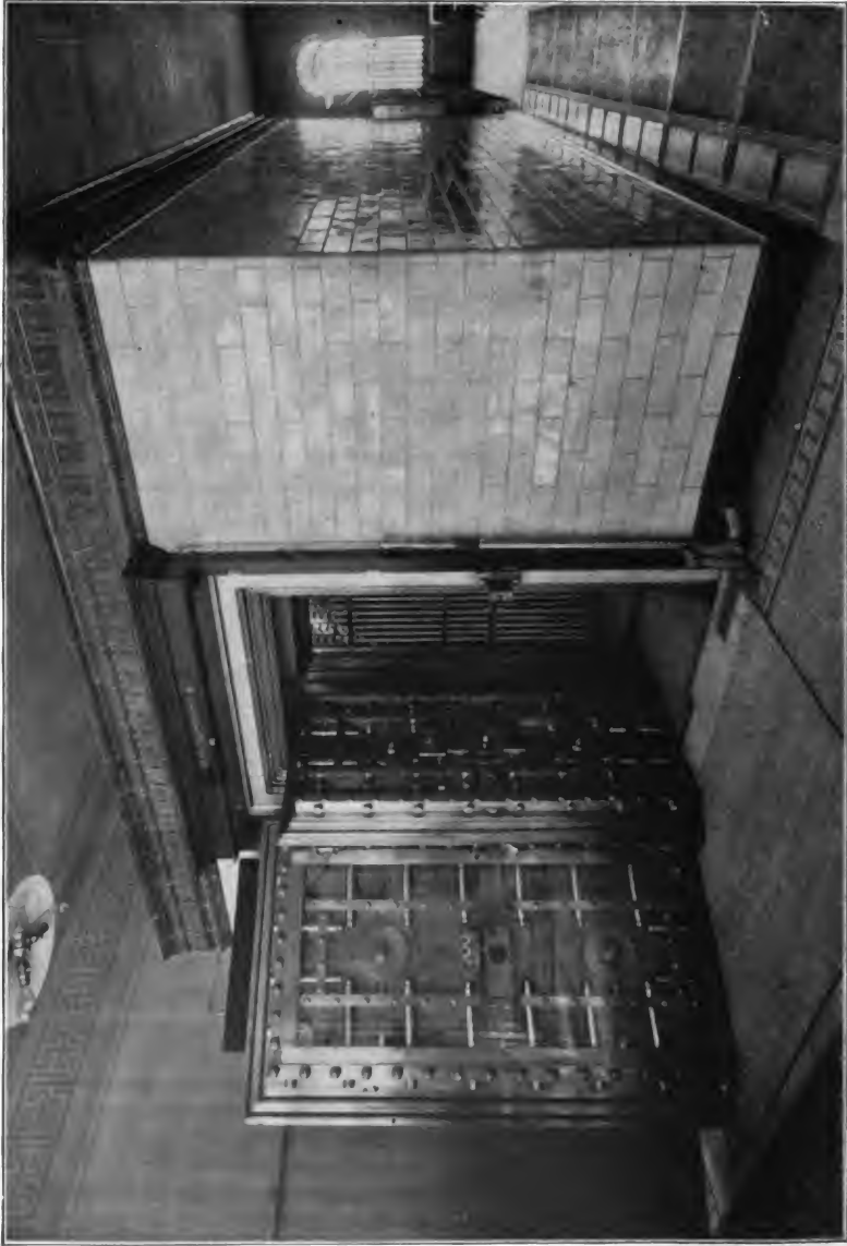
THE VAULT - PORTLAND TRUST CO., PORTLAND, ME.
